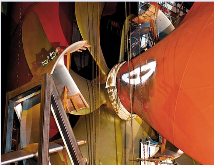
Becker's service team assisting the yard to minimise installation time
